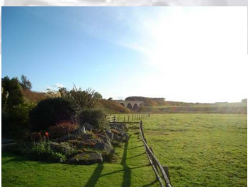
(above) Railway bridge over the Ythan river at Ellon
