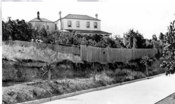
(above) Photo of Myrnong in Kooyong Road. The stables were to the right of the building.
